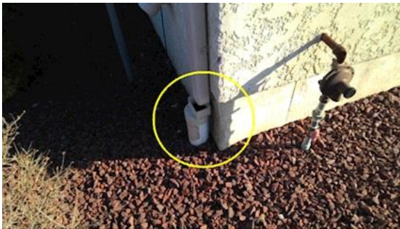
GUTTERS/DOWN SPOUTS: A simple repair with a gutter sleeve is recommended.
