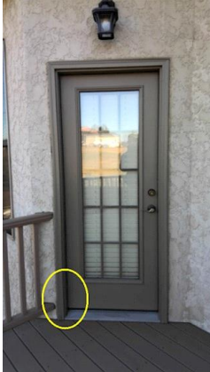
EXTERIOR DOORS: Molding deteriorated from moisture.
