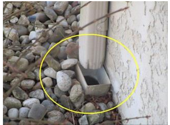
GUTTERS/DOWN SPOUTS: A simple repair with a gutter sleeve is recommended.
