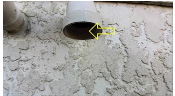
DRAFT CONTROL/VENT: No pest excluder screens.
