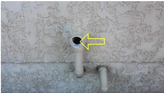
DRAFT CONTROL/VENT: No pest excluder screens.
